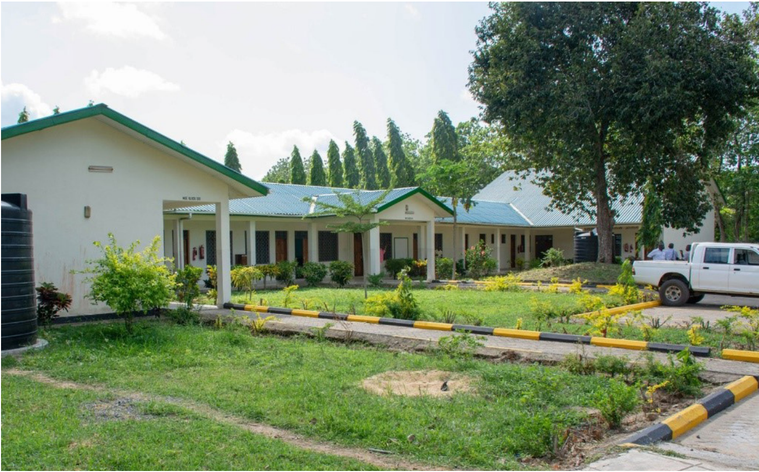
Mtwapa Energy Centre, Mombasa County
