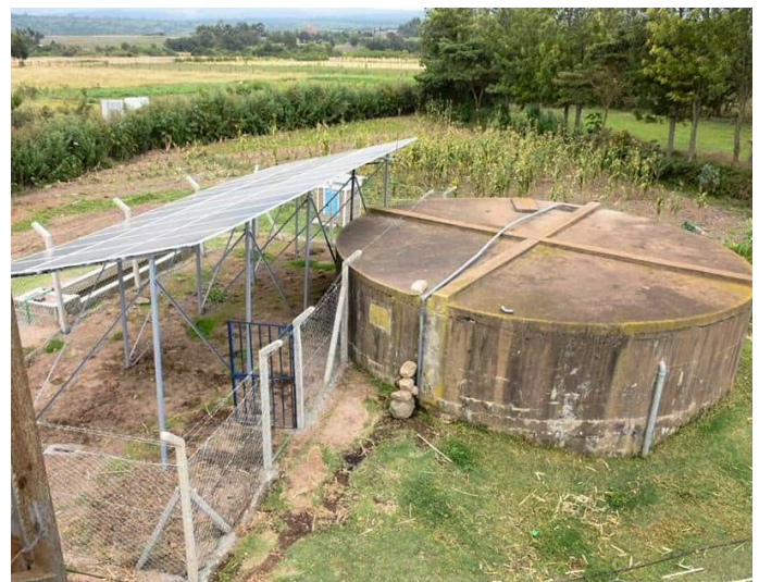
The solar powered borehole in Naromoru - Kiamathaga ward in Nyeri County.
